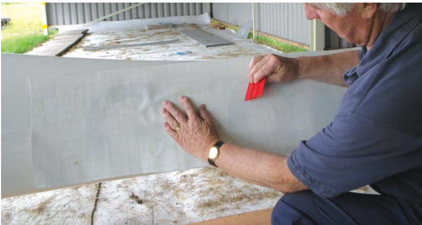
Final rub down using backing paper to protect
